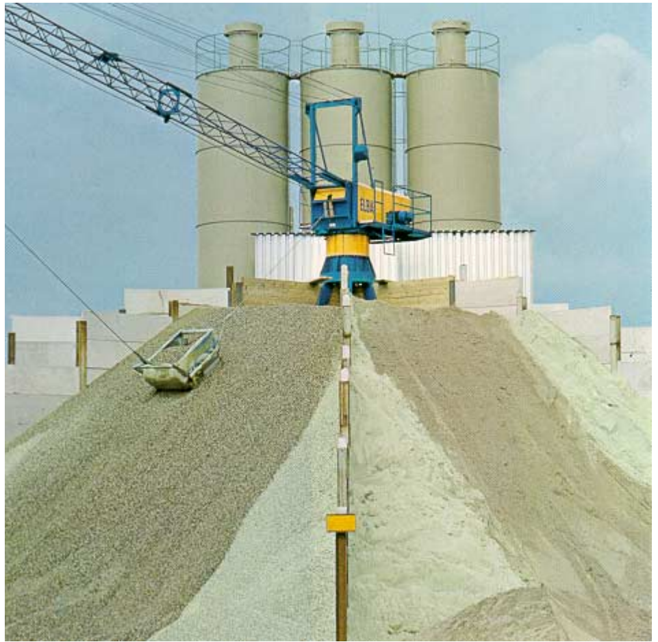
Fig. 26.11 Three-phase geared motor of various mounting on a scraper in a concrete mixing plant.
