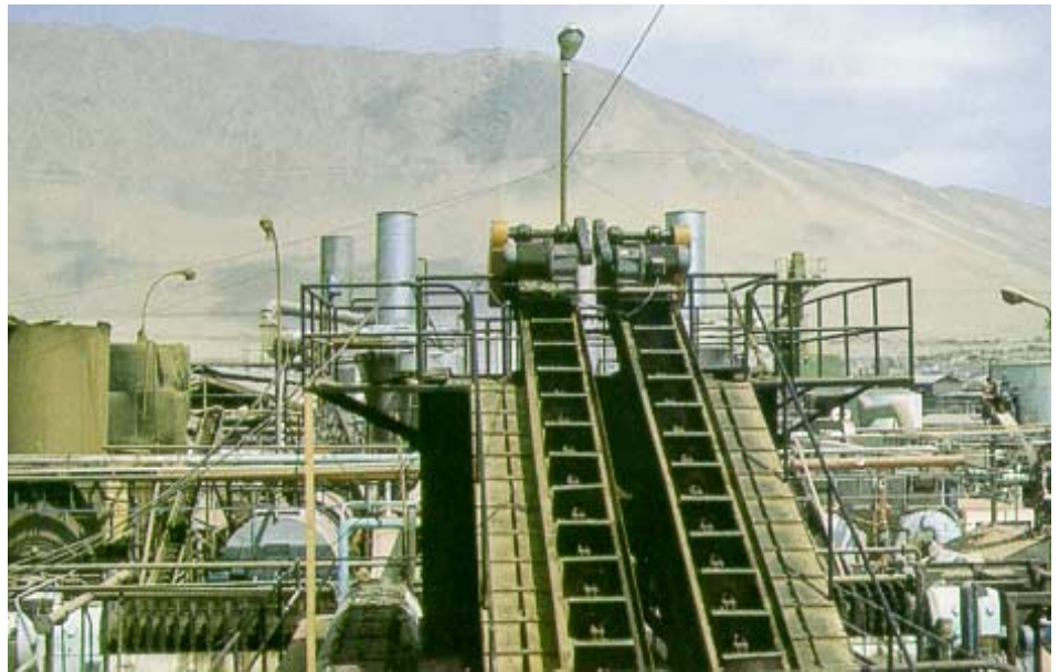
Fig. 26.34 Drives for rising conveyor belts in a dry, dusty atmosphere.
