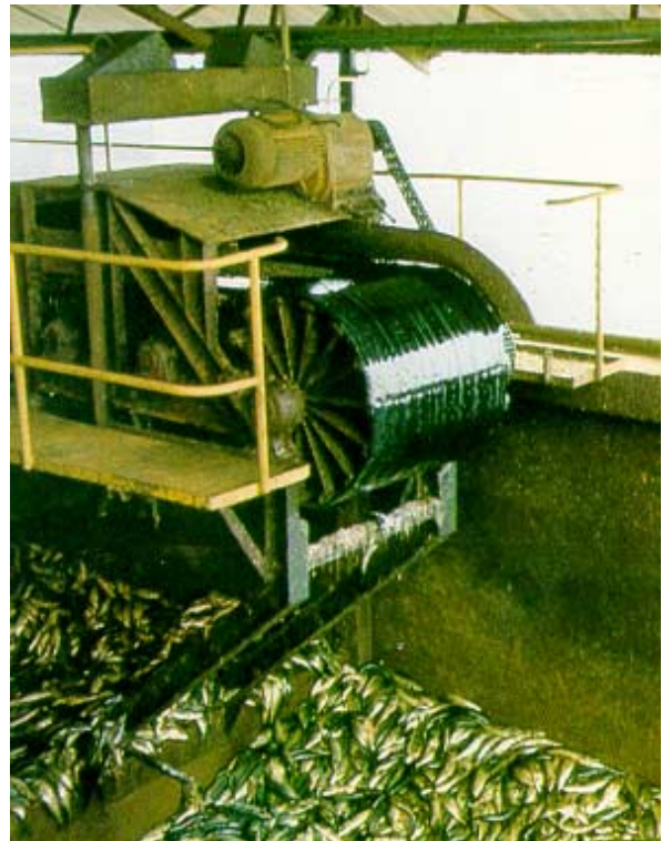
Fig. 26.32 Conveyor drive for saltwater fish.
