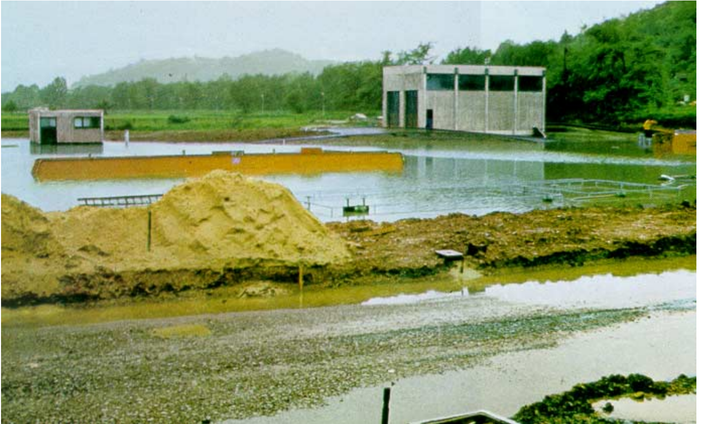
Fig. 26.30 Flooding of an aeration pond. The geared motors in the IP65 range, installed at the interceptor bridges have withstood this “test” extraordinarily well. Here the special degree of protection IP66 offer a real »chance of survival«.
