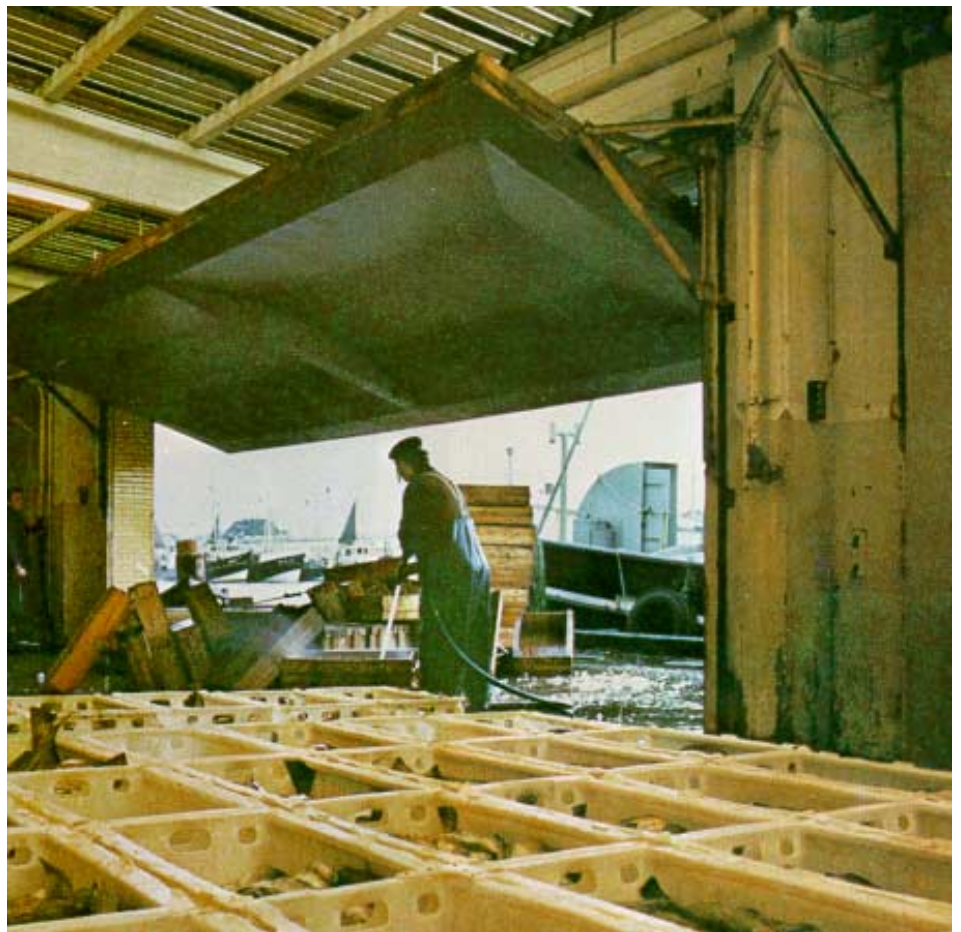
Fig. 26.23 Motor drive for a swing door in a fish auction hall with salty atmosphere.
