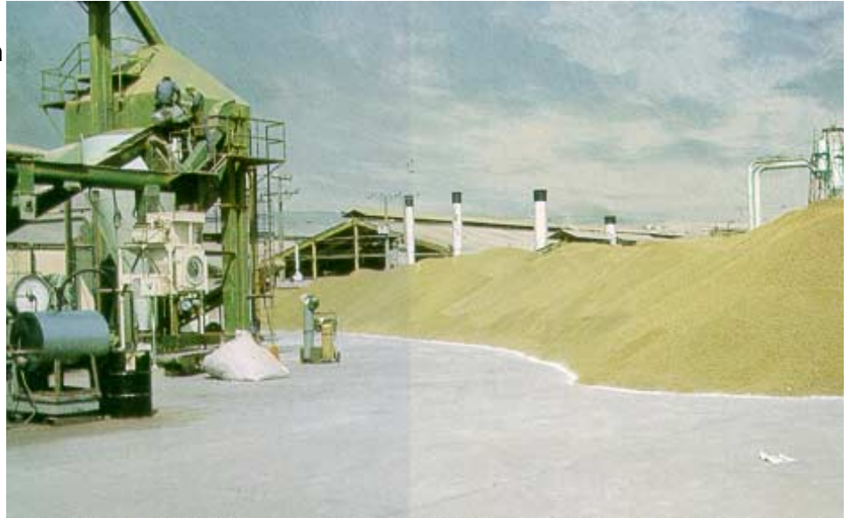
Fig. 26.33 Open-air installation in South America.
