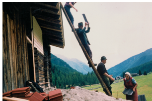
Figure 1.1.4 “Conveying system” for flat tiles, seen in South Tirol
